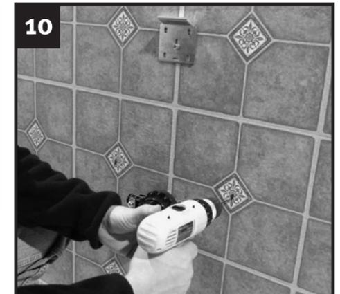
**10** Drill two more holes for the bracket and install additional screws. Also drill holes for the lower anchor screws.
