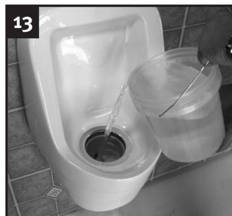
**13** Perform water test to ensure good flow and verify there are no leaks.
